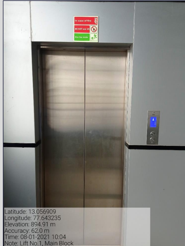
Lift in Main Block
