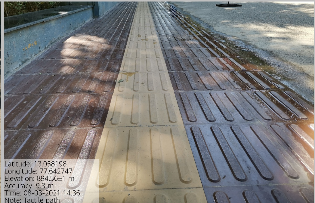
Tactile Path Leading to Main Block Entrance
