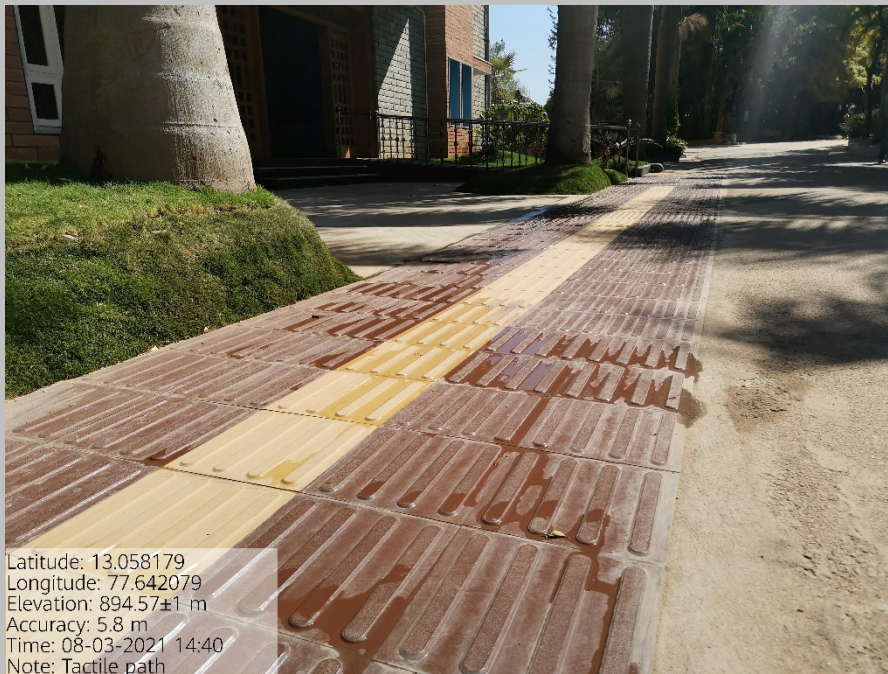
Tactile Path Leading to PG Block Entrance
