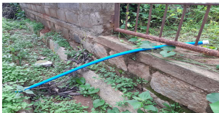
Direct Kauvery water pipeline connection given to the residents.
